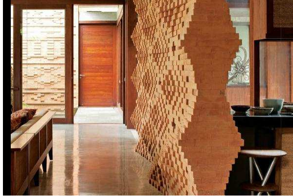
Brick separation wall in a Villa in Bali, Indonesia
