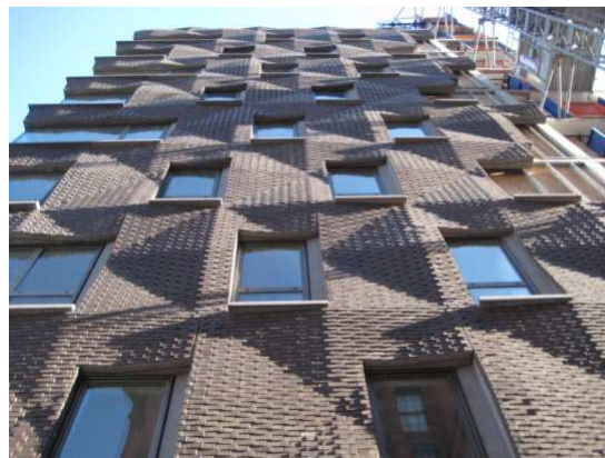
Brick facade, Apartment building, New York, USA
