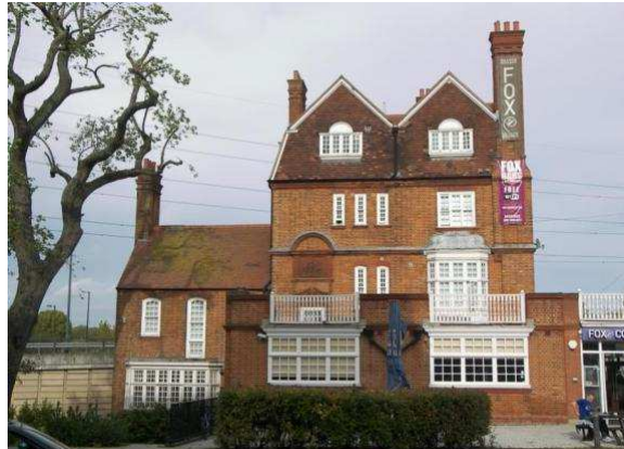
Bicklaying – Brick facades
